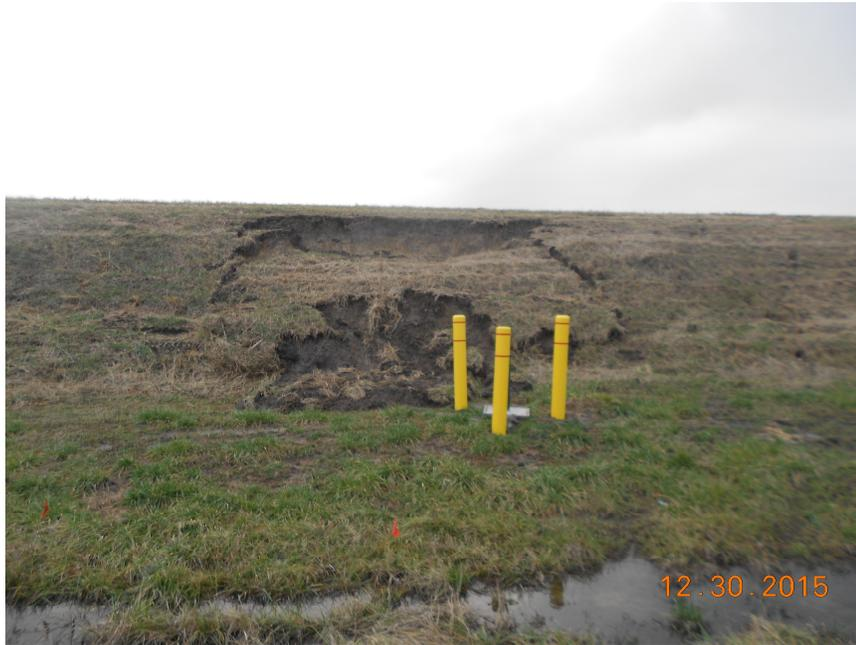
**Figure G.1. Photo of 2015 sloughing prior to repairs.**
