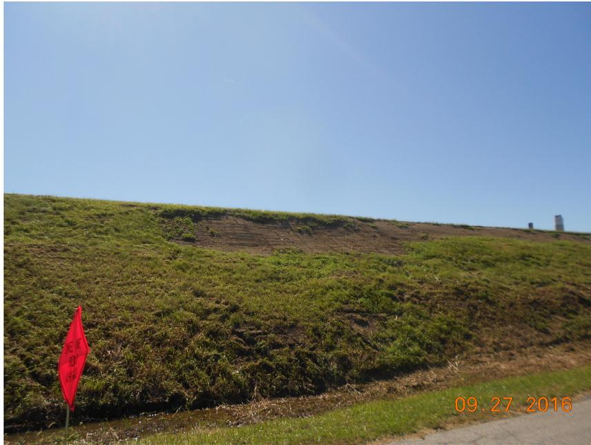
**Figure G.3. Photo of 2015 sloughing area after repairs.**
