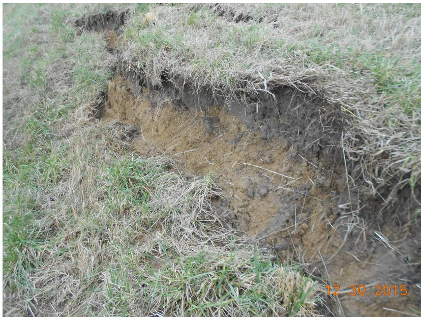
**Figure G.2. Photo of 2015 sloughing prior to repairs.**
